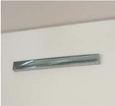
INDULSNAP plenum box with dust protection in the completed drywall. The extended neck protrudes beyond the wall structure, because it must still be equipped with acoustic elements.
