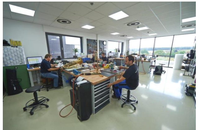
Comfort ceiling fan coil system INDULVENT ec and ceiling air diffuser INDULCLIP-ZA in the workshop area
