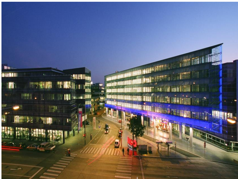
EURO PLAZA Vienna, building phase 4
