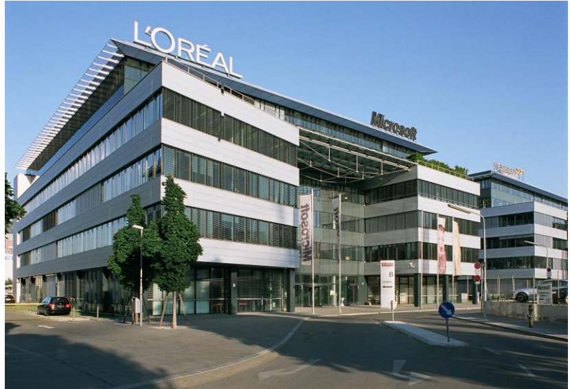
EURO PLAZA Vienna, building phase 1
