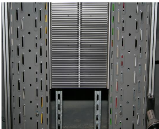
Details of visible installation Individual INDUCOOL-Compact elements with cable trays on both sides and strip luminaires.
