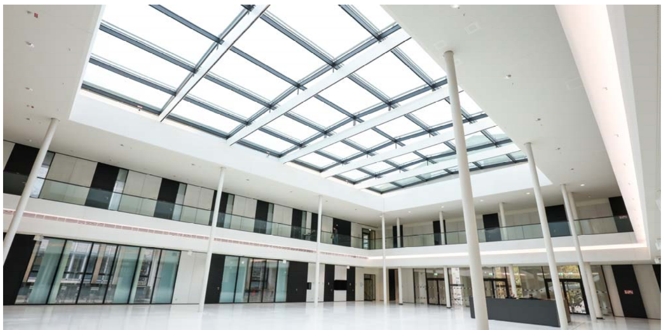
Portico hall with INDUL AV 45 diffusers discreetly arranged around the circumference of the hall.
