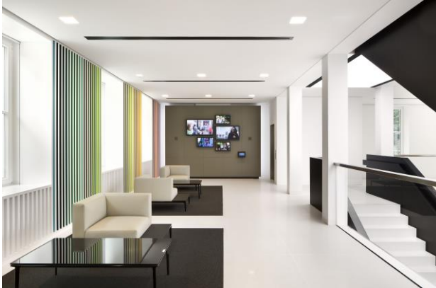
INDUL Linear diffusers in single structure integrated harmoniously and elegant in the ceiling design.
