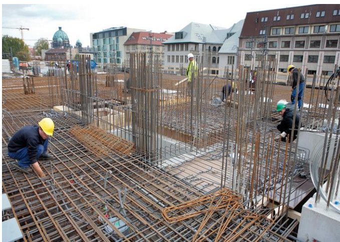
Installing reinforcement
