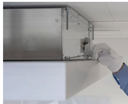
Figure 3: Undoing the nuts (M8).
