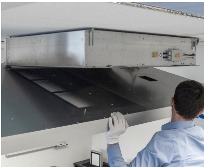
Figure 4: Opening the acoustic sail.
