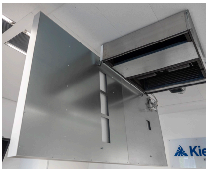
Figure 2: Pivoting of the lighting sail ensures ease of access for maintaining and inspecting the unit (VDI 6022).
