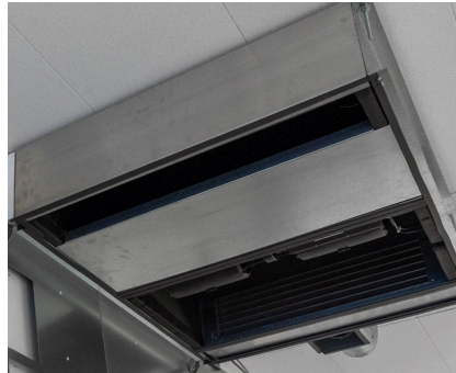
Figure 5: Access hatch for fan and heat exchanger.
