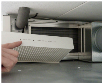
Figure 1: Inserting the filter cell (available as a spare part).
