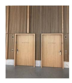
They are located in the 20.5 cm thick lightweight walls of the seminar rooms on the first and second floors, which have been designed to a particularly high standard. These partition walls feature vertical wooden slats of solid oak on the outside, into which the transfer slits are inconspicuously integrated. To achieve this, Kiefer manufactured transfer grilles with an extralong "neck", to bridge the width of the wall to the corridor side.
