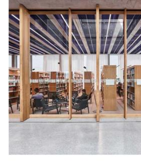
The corridor walls of the lecture halls on the first and second floors are made of fine oak slats. The openings of the INDUSILENT transfer grilles are also integrated into the vertical structure.
